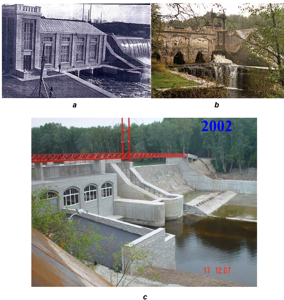
Fig. 3. Linnamäe hydropower plant: a – after commissioning in 1924; b – before restoration in 2001; c – after commissioning in 2002.
