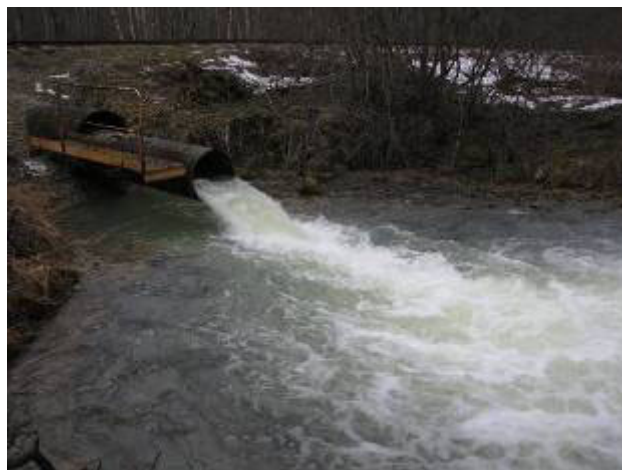
Fig. 5. Outflow from Aru-Lõuna limestone quarry.
